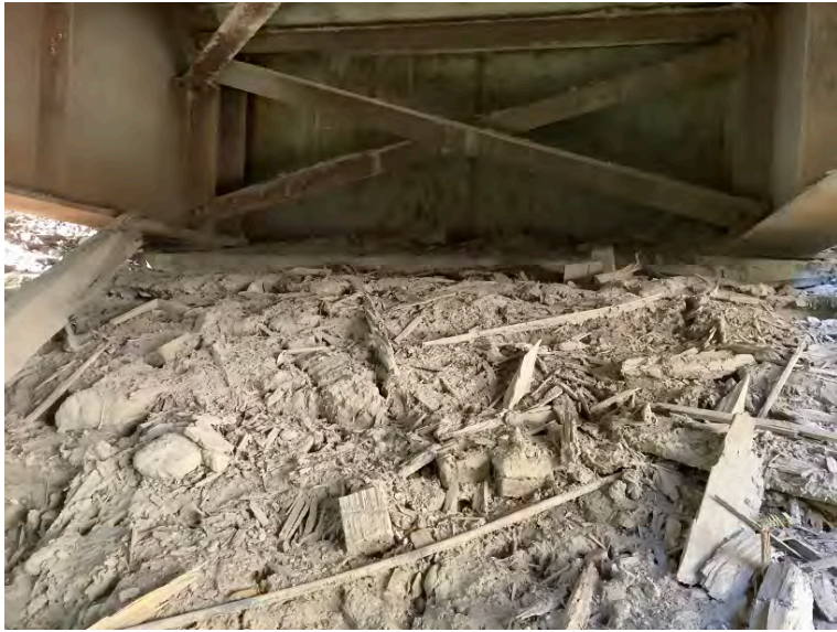
Right Bank Abutment when facing downstream
